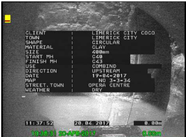
Photo: 41_41_259_A.jpg, 00:00:00 0m, Start node type, manhole, reference number : C 40
