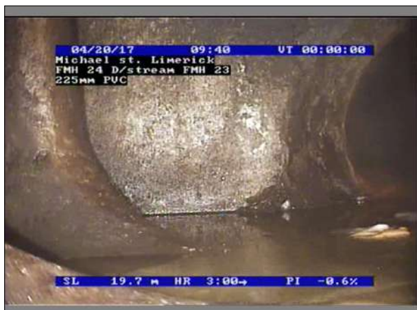
Photo: 5_5_31_A.jpg, 00:02:38 19.7m, Water level, 5% of the vertical dimension
