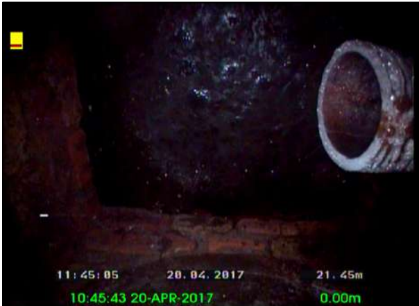
Photo: 41_41_271_A.jpg, 00:07:12 21.45m, General remark Remarks: BURIED MANHOLE CHAMBER
