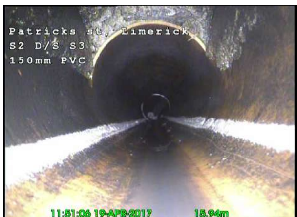
Photo: 32_32_189_A.jpg, 00:02:11 15.94m, Water level, 5% of the vertical dimension
