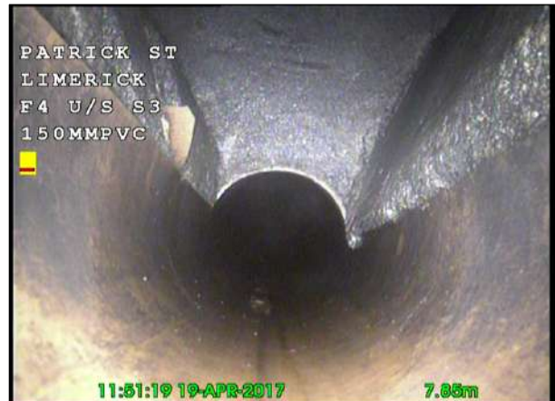
Photo: 25_25_153_A.jpg, 00:02:17 7.83m, Water level, 5% of the vertical dimension
