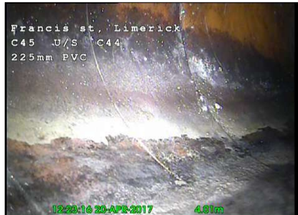
Photo: 42_42_283_A.jpg, 00:00:33 4.01m, Line deviates right
