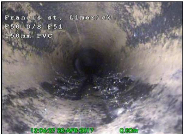
Photo: 44_44_290_A.jpg, 00:00:01 0m, Start node type, manhole, reference number : F 50
