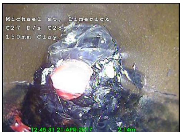
Photo: 46_46_303_A.jpg, 00:00:43 2.14m, Other obstacles, other object in invert, from 12 to 12 o'clock, 95% cross-sectional area loss Remarks: UNABLE TO PASS
