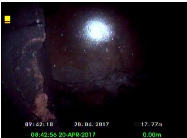
Photo: 33_33_199_A.jpg, 00:06:27 17.77m, Broken pipe, from 10 to 2 o'clock Remarks: PIPE ROOF BROKEN AND CAPPED
