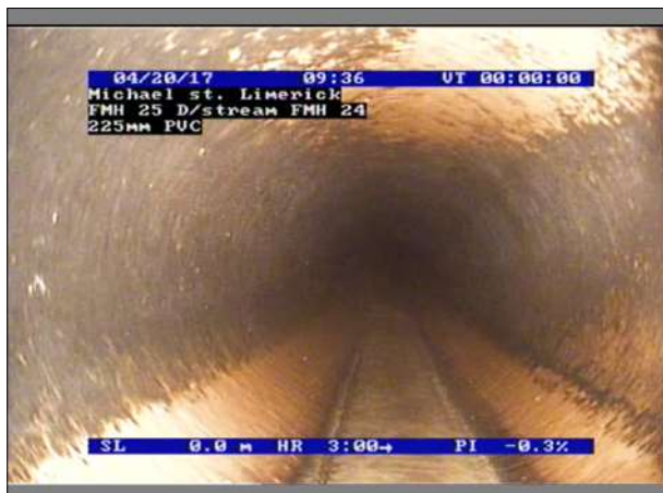
Photo: 4_4_4_A.jpg, 00:00:00 0m, Start node type, manhole, reference number : FMH 25
