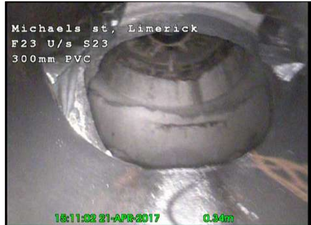
Photo: 48_48_310_A.jpg, 00:00:18 1m, Finish node type, manhole reference number: S 23
