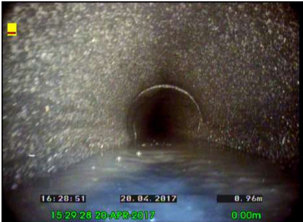
Photo: 38_38_237_A.jpg, 00:00:22 0.95m, Water level, 15% of the vertical dimension
