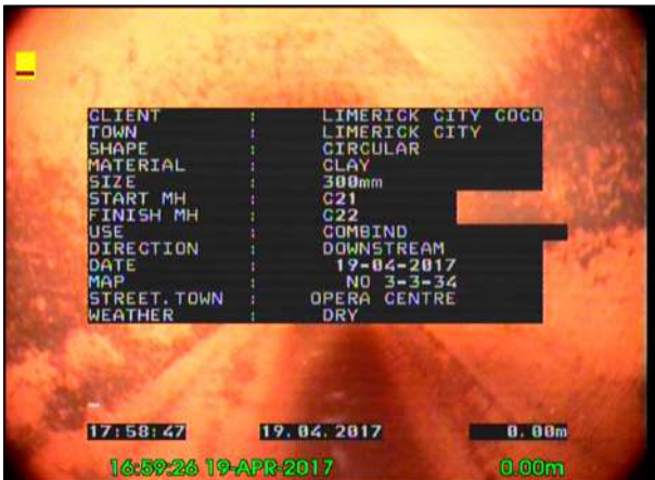
Photo: 21_21_128_A.jpg, 00:00:02 0m, Start node type, manhole, reference number : C 21
