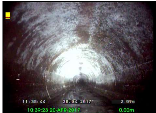
Photo: 41_41_260_A.jpg, 00:00:52 2.08m, Water level, 10% of the vertical dimension
