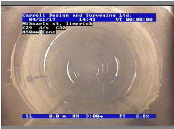
Photo: 15_15_15_A.jpg, 00:00:00 0m, Start node type, manhole, reference number : C29
