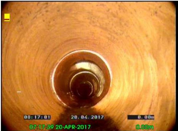
Photo: 35_35_214_A.jpg, 00:00:04 0m, Start node type, manhole, reference number : C 2
