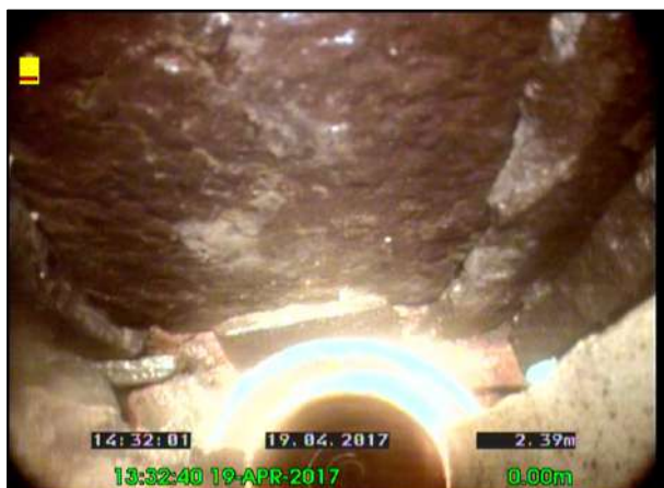
Photo: 16_16_60_A.jpg, 00:02:28 2.5m, General remark Remarks: CHAMBER
