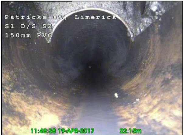
Photo: 31_31_184_A.jpg, 00:03:09 22.15m, Water level, 5% of the vertical dimension
