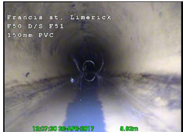
Photo: 44_44_292_A.jpg, 00:01:04 8.76m, Water level, 5% of the vertical dimension
