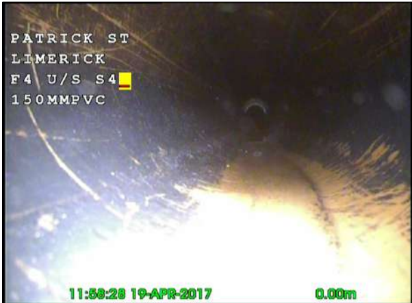
Photo: 26_26_155_A.jpg, 00:00:01 0m, Start node type, manhole, reference number : FMH 4
