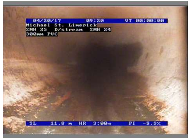
Photo: 1_1_18_A.jpg, 00:02:04 11.8m, Water level, 5% of the vertical dimension
