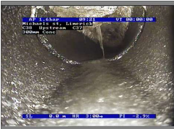
Photo: 8_8_8_A.jpg, 00:00:00 0m, Start node type, manhole, reference number : C38
