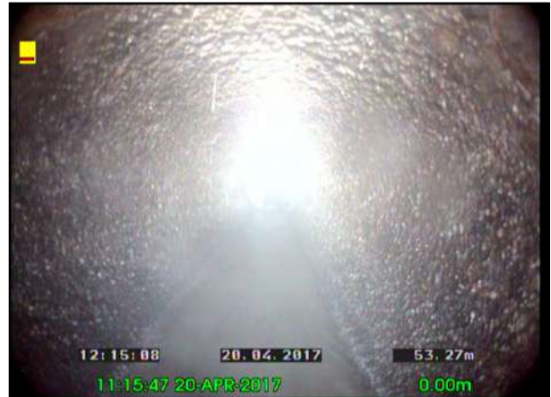
Photo: 39_39_254_A.jpg, 00:10:26 53.27m, Shape changes to circular, 300mm high Remarks: ??????
