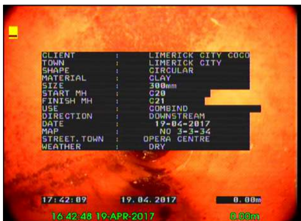
Photo: 20_20_110_A.jpg, 00:00:01 0m, Start node type, manhole, reference number : C 20
