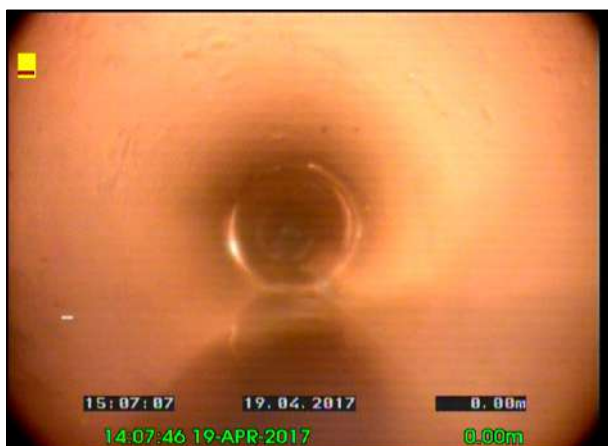
Photo: 17_17_82_A.jpg, 00:00:01 0m, Start node type, manhole, reference number : C 4
