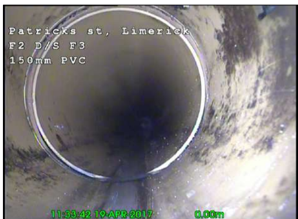
Photo: 29_29_169_A.jpg, 00:00:02 0m, Start node type, manhole, reference number : FMH 2
