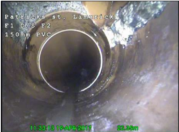
Photo: 28_28_167_A.jpg, 00:03:40 23.35m, Water level, 5% of the vertical dimension
