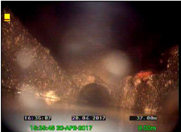
Photo: 38_38_241_A.jpg, 00:05:01 37m, Water level, 15% of the vertical dimension
