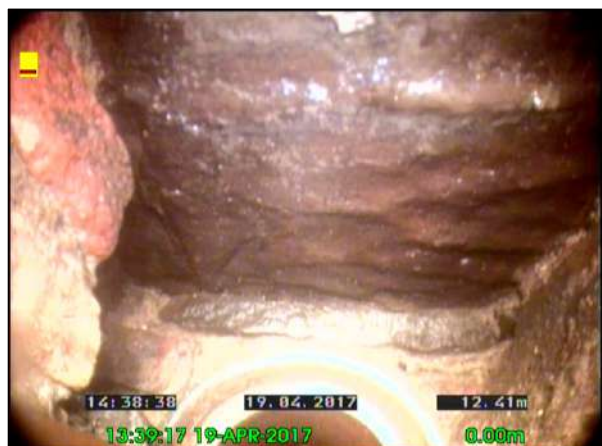
Photo: 16_16_66_A.jpg, 00:08:36 12.41m, General remark Remarks: CHAMBER
