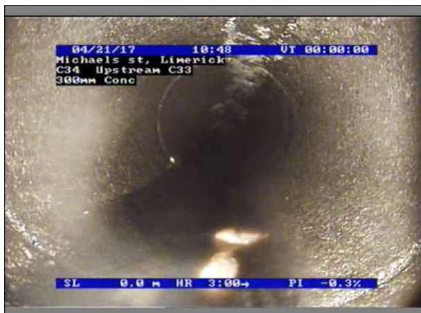
Photo: 11_11_11_A.jpg, 00:00:00 0m, Start node type, manhole, reference number : C34
