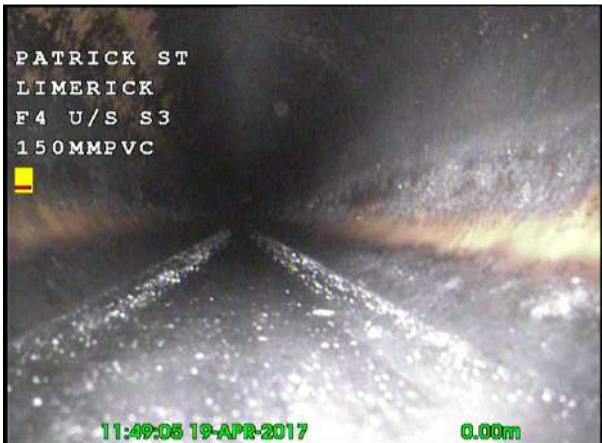
Photo: 25_25_151_A.jpg, 00:00:04 0m, Start node type, manhole, reference number : FMH 4
