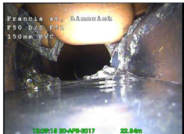
Photo: 44_44_295_A.jpg, 00:02:51 22.84m, Finish node type, manhole reference number: F 51
