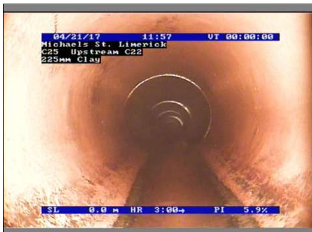
Photo: 12_12_12_A.jpg, 00:00:00 0m, Start node type, manhole, reference number : C25
