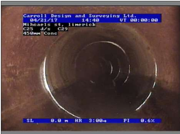
Photo: 14_14_14_A.jpg, 00:00:00 0m, Start node type, manhole, reference number : C25
