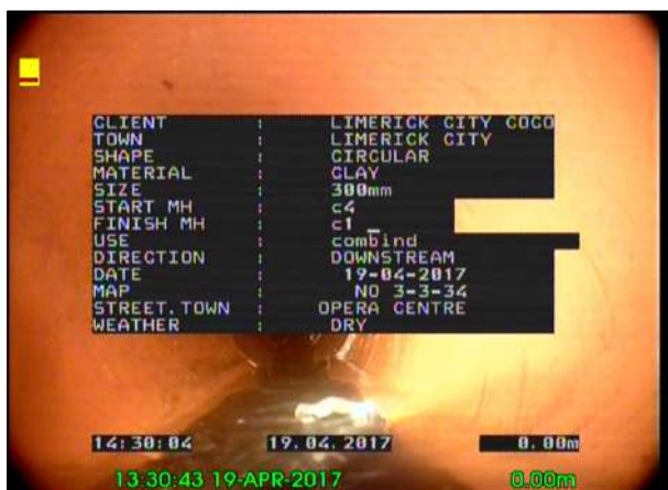
Photo: 16_16_57_A.jpg, 00:00:02 0m, Start node type, manhole, reference number : C 4
