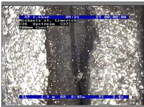
Photo: 8.8_37_A.jpg, 00:00:46 1.9m, Open joint, medium
