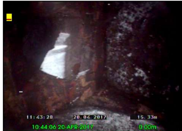
Photo: 41_41_268_A.jpg, 00:05:36 15.33m, General remark Remarks: BURIED MANHOLE CHAMBER ON LINE
