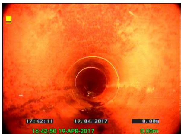
Photo: 20_20_111_A.jpg, 00:00:01 0m, Water level, 5% of the vertical dimension
