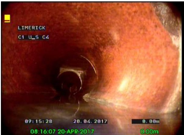
Photo: 34_34_205_A.jpg, 00:00:00 0m, Start node type, manhole, reference number : C 1
