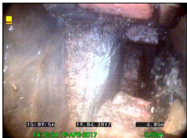
Photo: 17_17_86_A.jpg, 00:02:55 4.05m, General remark Remarks: CHAMBER
