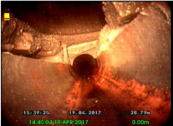
Photo: 18_18_106_A.jpg, 00:05:12 28.78m, Water level, 5% of the vertical dimension
