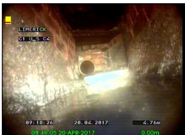
Photo: 34_34_212_A.jpg, 00:02:58 4.76m, Water level, 5% of the vertical dimension
