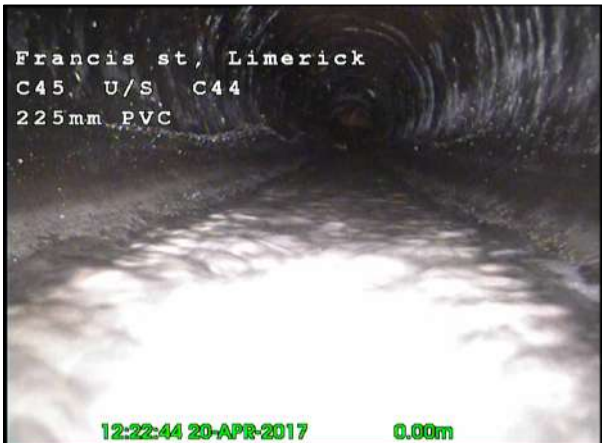
Photo: 42_42_281_A.jpg, 00:00:01 0m, Start node type, manhole, reference number : C 45
