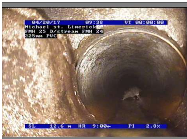
Photo: 4_4_27_A.jpg, 00:01:25 12.6m, Water level, 5% of the vertical dimension
