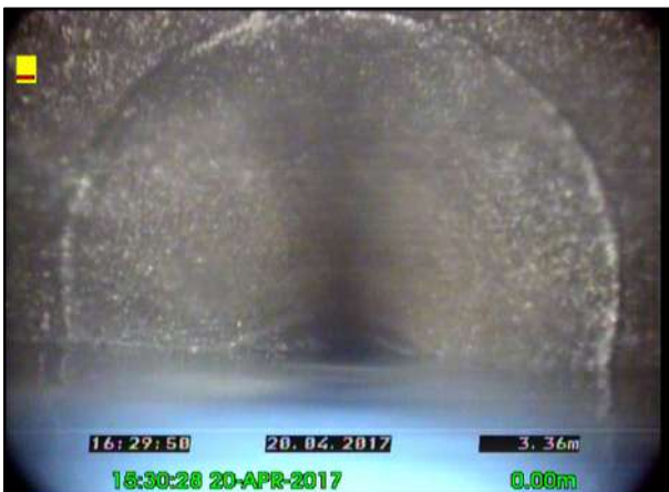
Photo: 38_38_239_A.jpg, 00:01:21 3.35m, Water level, 30% of the vertical dimension
