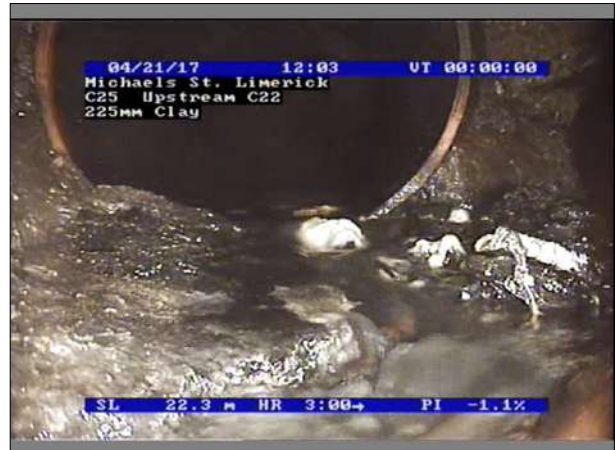
Photo: 12_12_54_A.jpg, 00:05:50 22.3m, Water level, 5% of the vertical dimension
