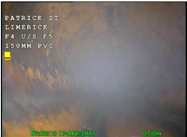
Photo: 24_24_146_A.jpg, 00:00:00 0m, Start node type, manhole, reference number : FMH 4
