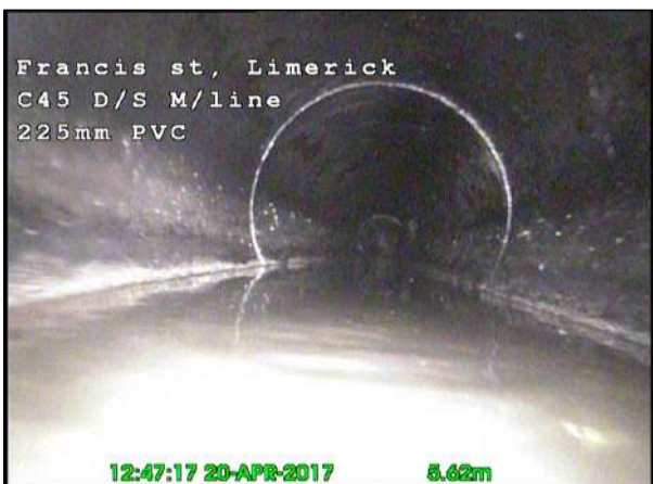
Photo: 43_43_287_A.jpg, 00:00:39 5.62m, Water level, 10% of the vertical dimension
