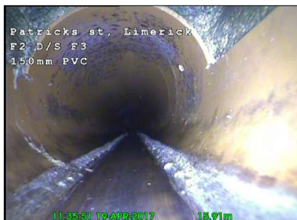
Photo: 29_29_173_A.jpg, 00:02:11 15.92m, Water level, 5% of the vertical dimension
