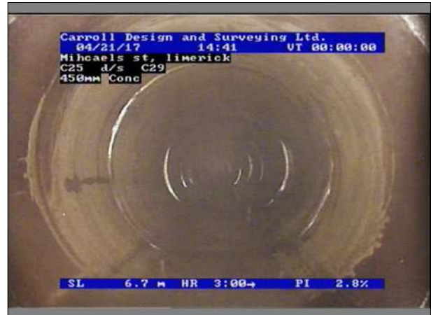
Photo: 14_14_318_A.jpg, 00:01:17 6.7m, Water level, 5% of the vertical dimension
