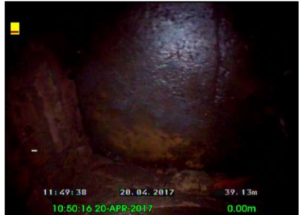
Photo: 41_41_277_A.jpg, 00:11:46 39.13m, General remark Remarks: BURIED MANHOLE CHAMBER
