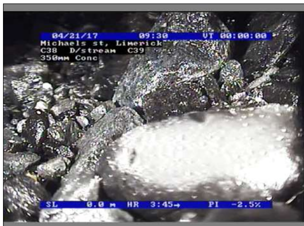
Photo: 9_9_9_A.jpg, 00:00:00 0m, Start node type, manhole, reference number : C38
