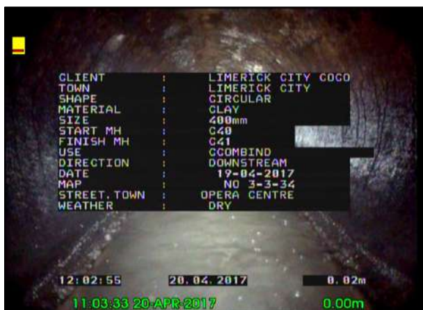
Photo: 39_39_243_A.jpg, 00:00:01 0m, Start node type, manhole, reference number : C 40
