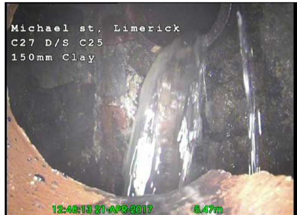
Photo: 45_45_299_A.jpg, 00:00:53 5.47m, Start node type, manhole, reference number : C 27
