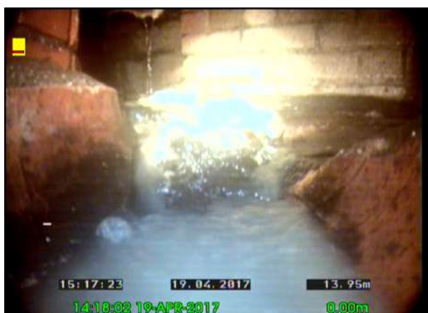
Photo: 17_17_99_A.jpg, 00:10:14 13.83m, Water level, 5% of the vertical dimension
