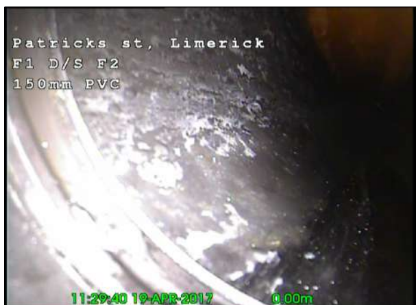
Photo: 28_28_162_A.jpg, 00:00:07 0m, Start node type, manhole, reference number : FMH 1
