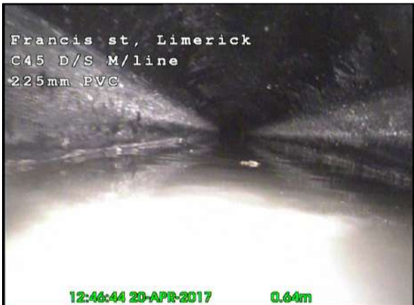
Photo: 43_43_285_A.jpg, 00:00:06 0.64m, Start node type, manhole, reference number : C 45
