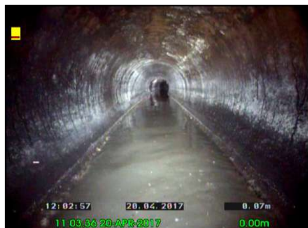
Photo: 39_39_244_A.jpg, 00:00:04 0.07m, Water level, 10% of the vertical dimension
