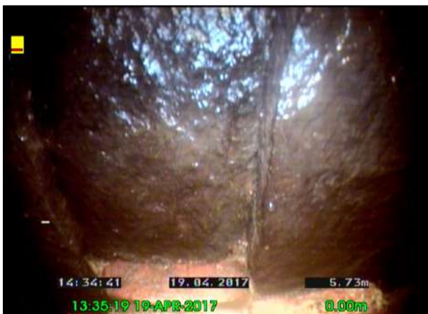
Photo: 16_16_62_A.jpg, 00:04:39 5.73m, General remark Remarks: CHAMBER
