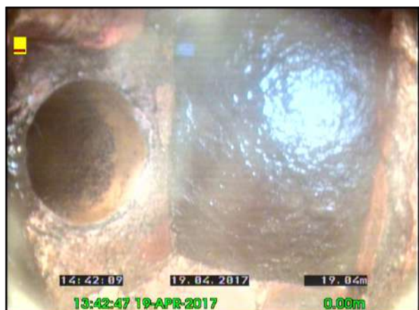
Photo: 16_16_72_A.jpg, 00:12:07 19.04m, General remark Remarks: CHAMBER
