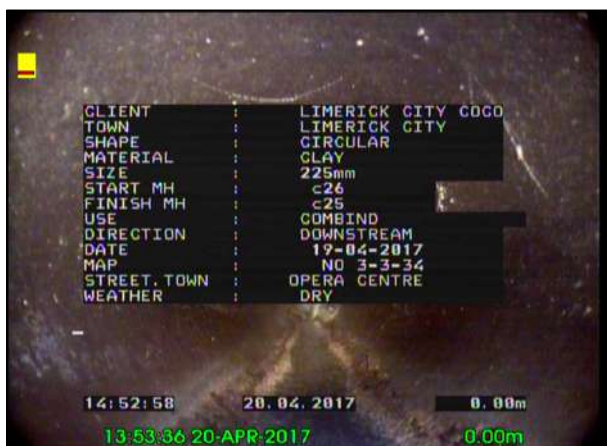
Photo: 37_37_230_A.jpg, 00:00:00 0m, Start node type, manhole, reference number : C 26
