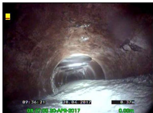
Photo: 33_33_194_A.jpg, 00:00:30 0.37m, Water level, 40% of the vertical dimension
