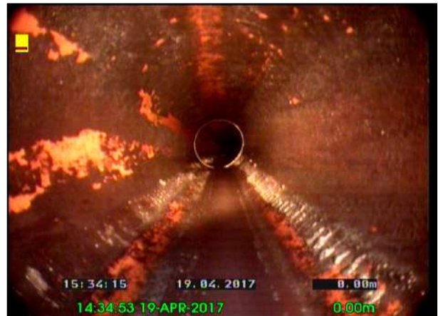
Photo: 18_18_102_A.jpg, 00:00:02 0m, Water level, 5% of the vertical dimension
