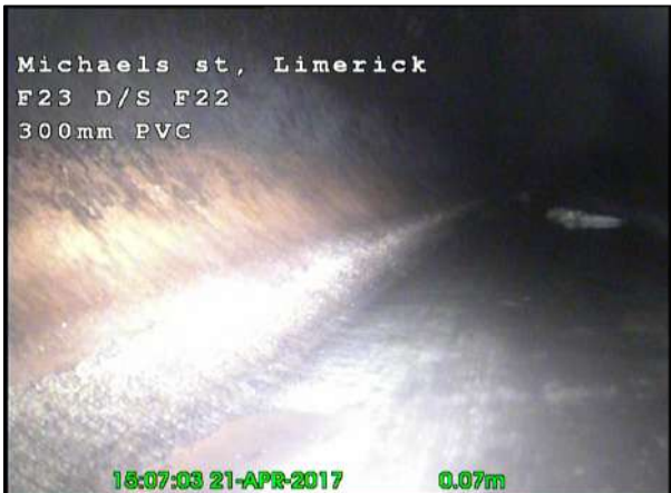
Photo: 47_47_304_A.jpg, 00:00:04 0m, Start node type, manhole, reference number : F 23
