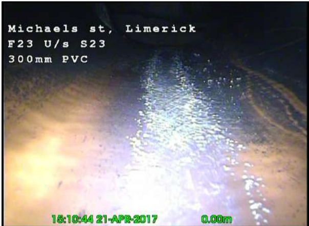
Photo: 48_48_308_A.jpg, 00:00:00 0m, Start node type, manhole, reference number : F 23
