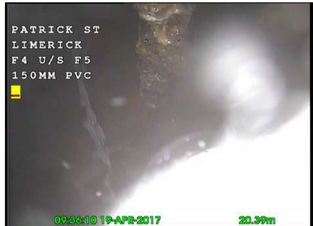
Photo: 24_24_148_A.jpg, 00:03:55 20.39m, Water level, 10% of the vertical dimension
