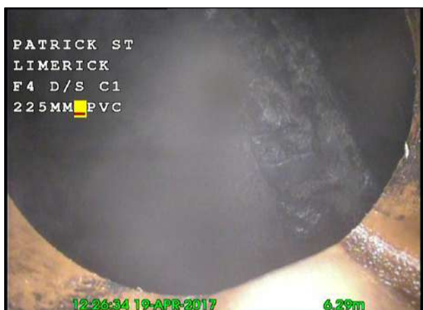
Photo: 23_23_144_A.jpg, 00:01:00 6.29m, Water level, 5% of the vertical dimension
