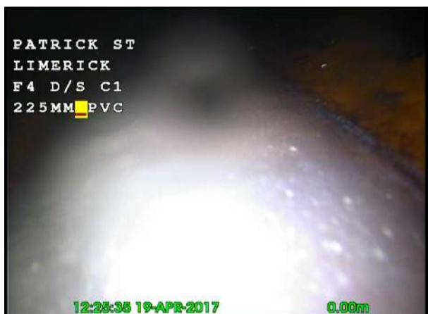
Photo: 23_23_142_A.jpg, 00:00:01 0m, Start node type, manhole, reference number : FMH 4
