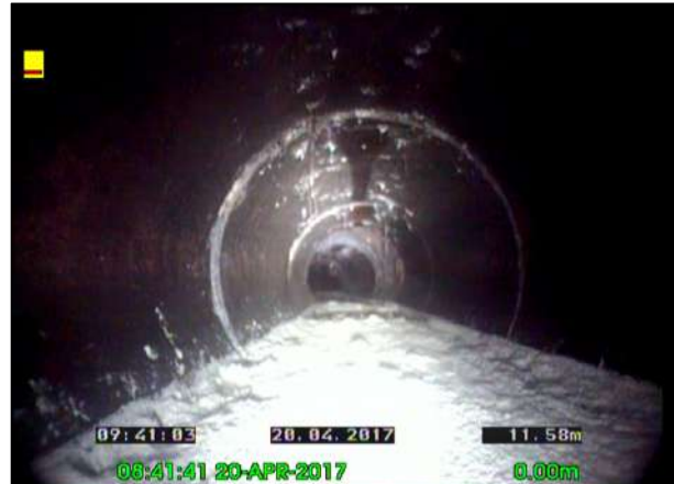
Photo: 33_33_197_A.jpg, 00:05:12 11.57m, Water level, 15% of the vertical dimension
