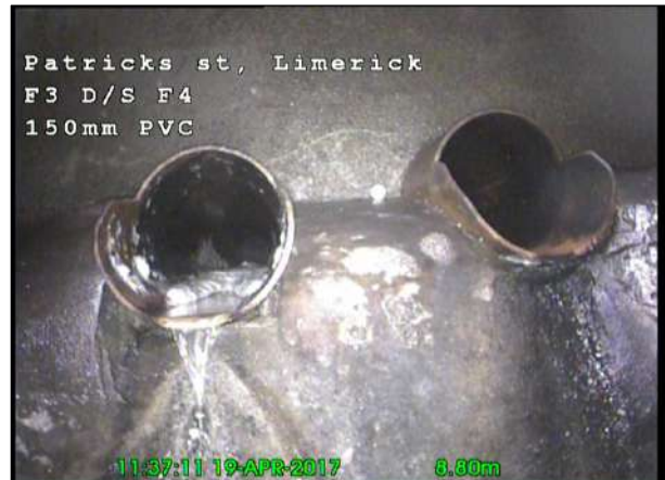
Photo: 30_30_178_A.jpg, 00:01:03 8.8m, Finish node type, manhole reference number: FMH 4
