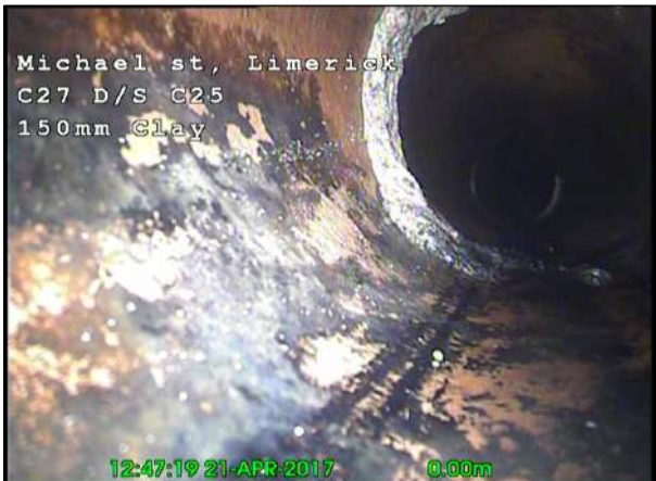
Photo: 45_45_296_A.jpg, 00:00:00 0m, Start node type, manhole, reference number : C 27
