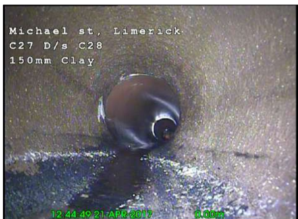
Photo: 46_46_300_A.jpg, 00:00:01 0m, Start node type, manhole, reference number : C 27
