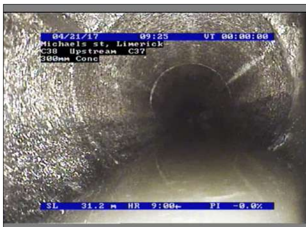
Photo: 8.8_39_A.jpg, 00:04:35 31.2m, Water level, 10% of the vertical dimension
