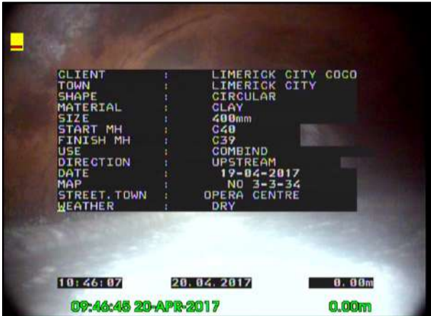
Photo: 40_40_257_A.jpg, 00:00:01 0m, Start node type, manhole, reference number : C 40
