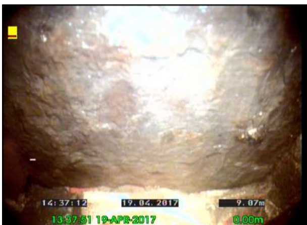
Photo: 16_16_65_A.jpg, 00:07:10 9.87m, General remark Remarks: CHAMBER
