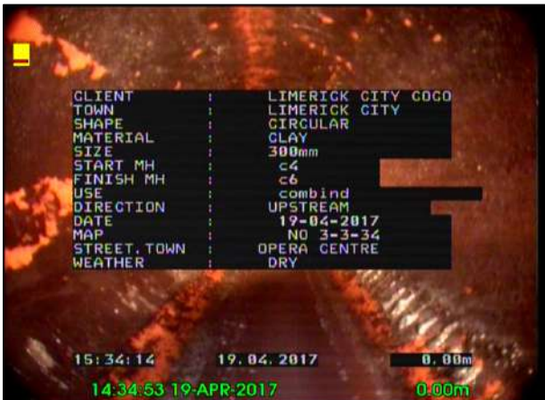
Photo: 18_18_101_A.jpg, 00:00:02 0m, Start node type, manhole, reference number : C 4
