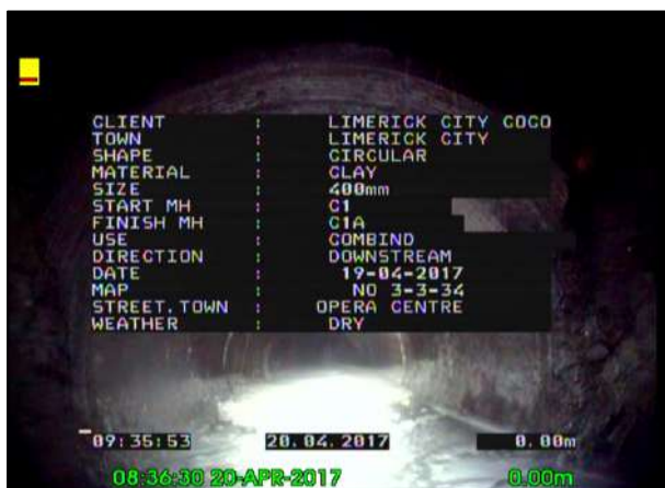
Photo: 33_33_191_A.jpg, 00:00:01 0m, Start node type, manhole, reference number : C 1
