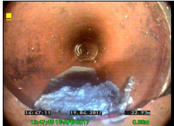
Photo: 16_16_81_A.jpg, 00:17:09 22.93m, Survey abandoned Remarks: UNABLE TO TRAVEL
