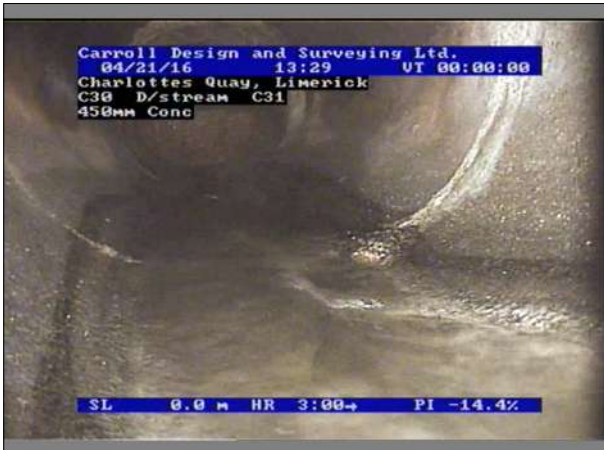
Photo: 13_13_13_A.jpg, 00:00:00 0m, Start node type, manhole, reference number : C30
