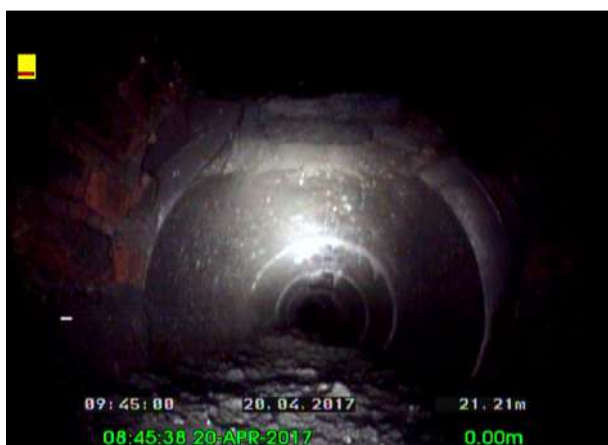
Photo: 33_33_203_A.jpg, 00:09:09 21.21m, General remark Remarks: CHAMBER
