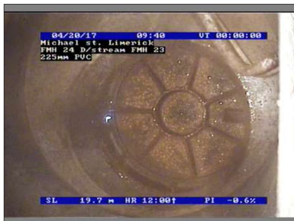
Photo: 5_5_32_A.jpg, 00:02:38 19.7m, Finish node type, manhole reference number: FMH 23
