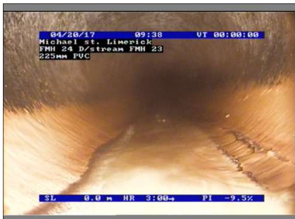
Photo: 5_5_5_A.jpg, 00:00:00 0m, Start node type, manhole, reference number : FMH 24
