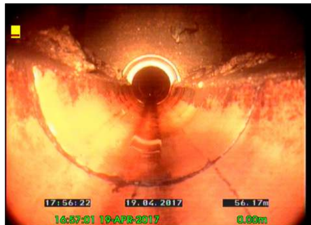
Photo: 20_20_126_A.jpg, 00:14:15 56.16m, Water level, 5% of the vertical dimension
