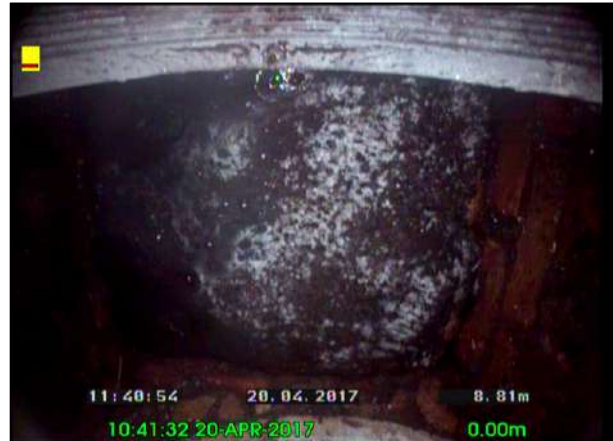
Photo: 41_41_264_A.jpg, 00:03:01 8.81m, General remark Remarks: BURIED MANHOLE CHAMBER ON LINE
